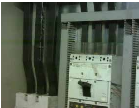
The middle rail requires inspection, because it is heating up to almost 80 degrees at some points.
