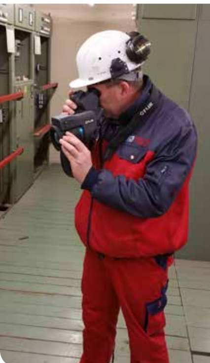
Martin Adler taking thermal images of a low-voltage main distribution
