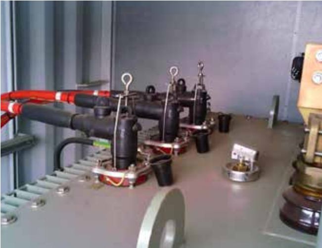
Alternator with abnormality on the primary front plug connector. A bent pin on the angle plug connector is found to be the cause.
