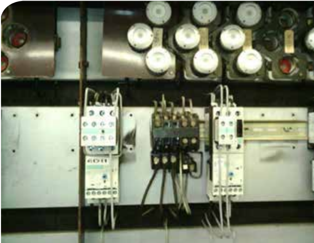
The middle phase of this motor protection switch looks abnormal. This could indicate increased resistance at the terminal connection.
