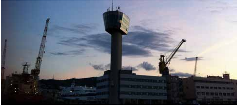
All activity of the port pilots is being coordinated and monitored from the control tower.
