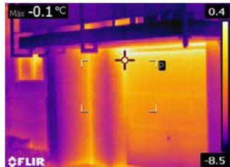
The tenant of this apartment complained about the permanently cold floor. The problem: The concrete slab of the balcony unintentionally served as a thermal bridge. Through the concrete slab, the apartment was therefore also heating the garage. The remedy consisted of insulating the garage ceiling from below.
